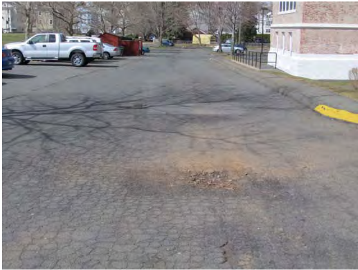
Asphalt paving exhibits areas of significant wear including alligatoring
