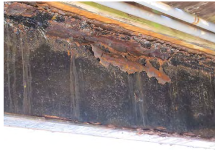
View of typical rust damage/steel deterioration on steel framing at underside of bridge
