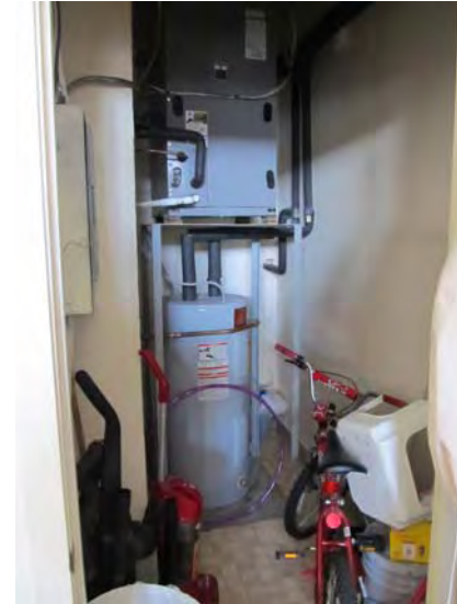
Typical in-unit air handler component of heat pump system and freestanding electric domestic hot water tank
