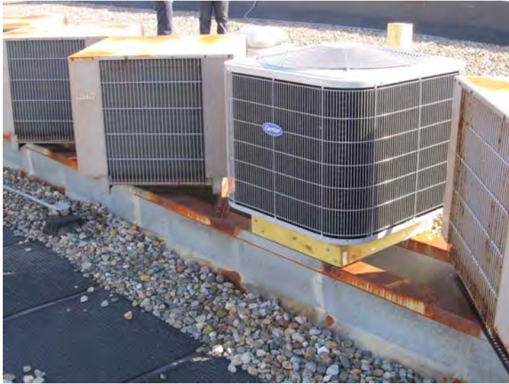
Rooftop-mounted condensers for heat pump systems that serve in-unit heating/cooling needs – Note all but seven condensers date to the 1985 renovation
