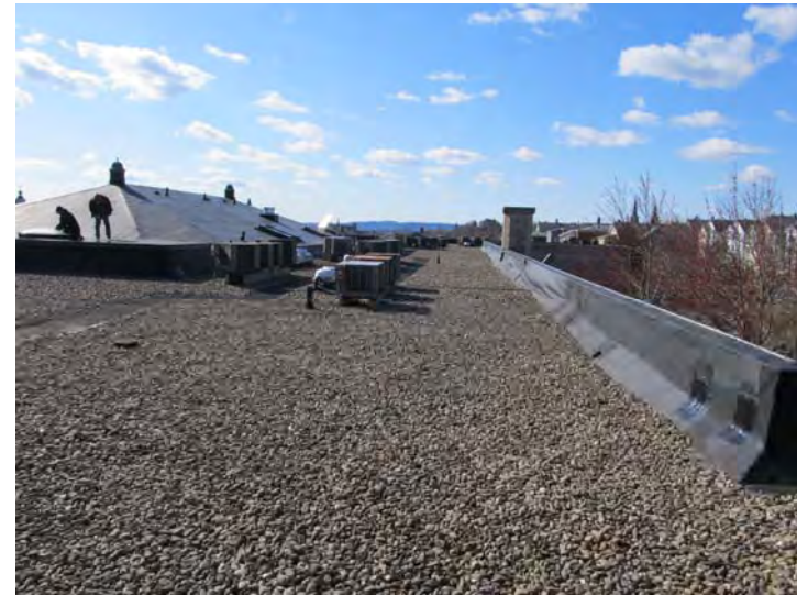
Roof coverings date to the 1985 renovation – Minor repair work ongoing at time of assessment
