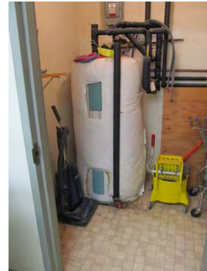
Typical electric-type domestic hot water tank serving a common laundry room
