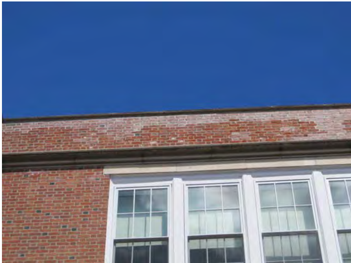
Isolated areas of worn brick and/or missing mortar in brickwork noted
