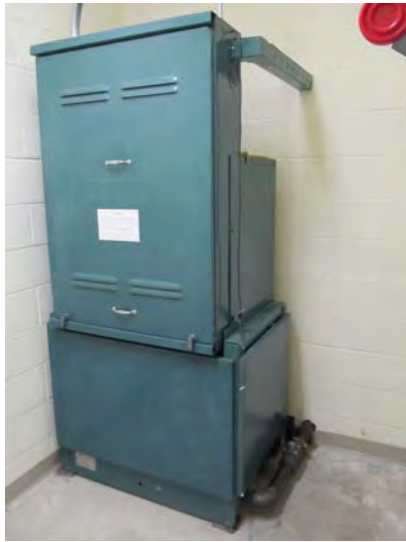
Original hydro-mechanical and controller/dispatcher unit for elevator – Equipment maintained under terms of a full service contract
