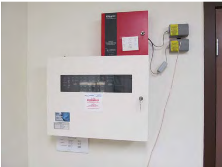
Original zone-type fire alarm control panel
